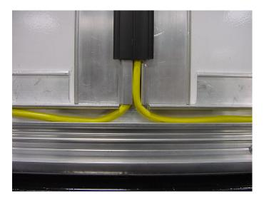
Figure 7-7 Picture of Joining Trim Cutout where Joining Trim enters Ramp Trim
